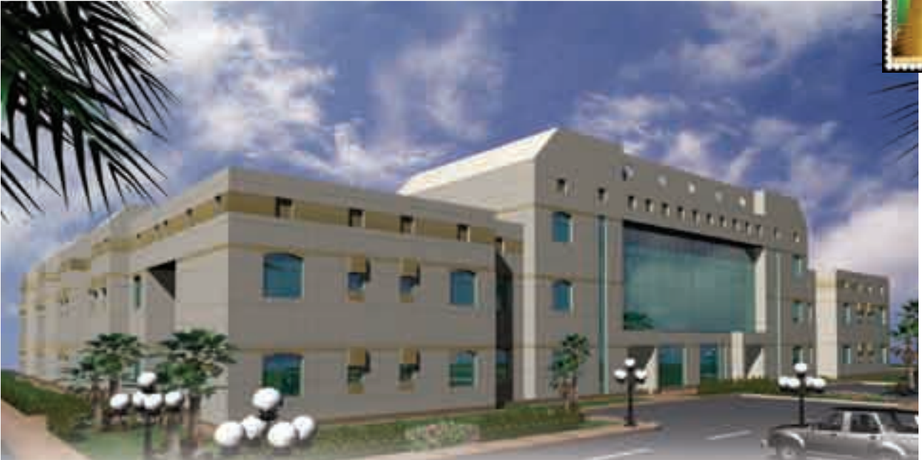
Building of Prince Salman Handicapped Children Center at Hail
