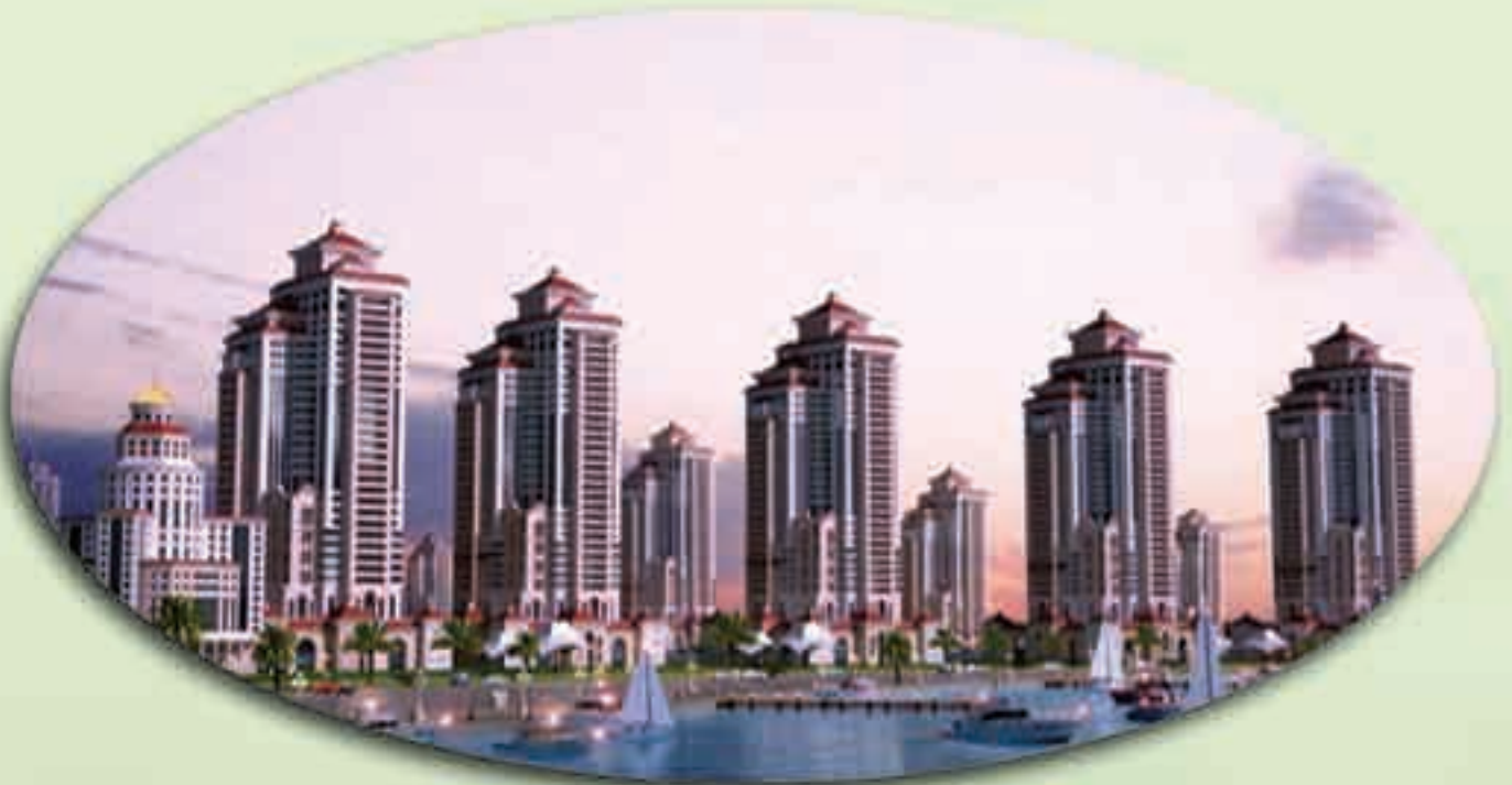
Waterfront tower project of Nujoom Islands
