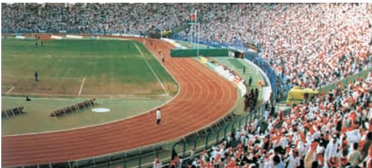
One of the corners of King Fahad International Stadium
